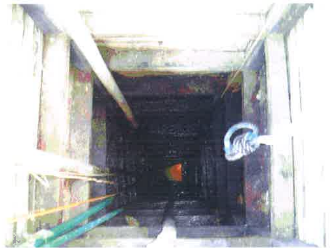
Figure 4. A shaft used by local gold miners for extracting gold ore at Cineam area
